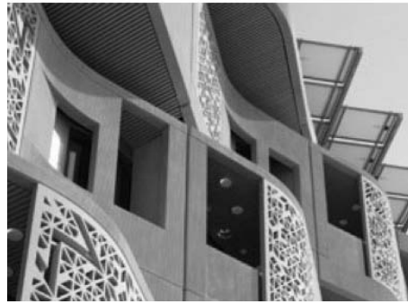
Fig. 1 The concrete facade of a building at the Masdar Institute.
