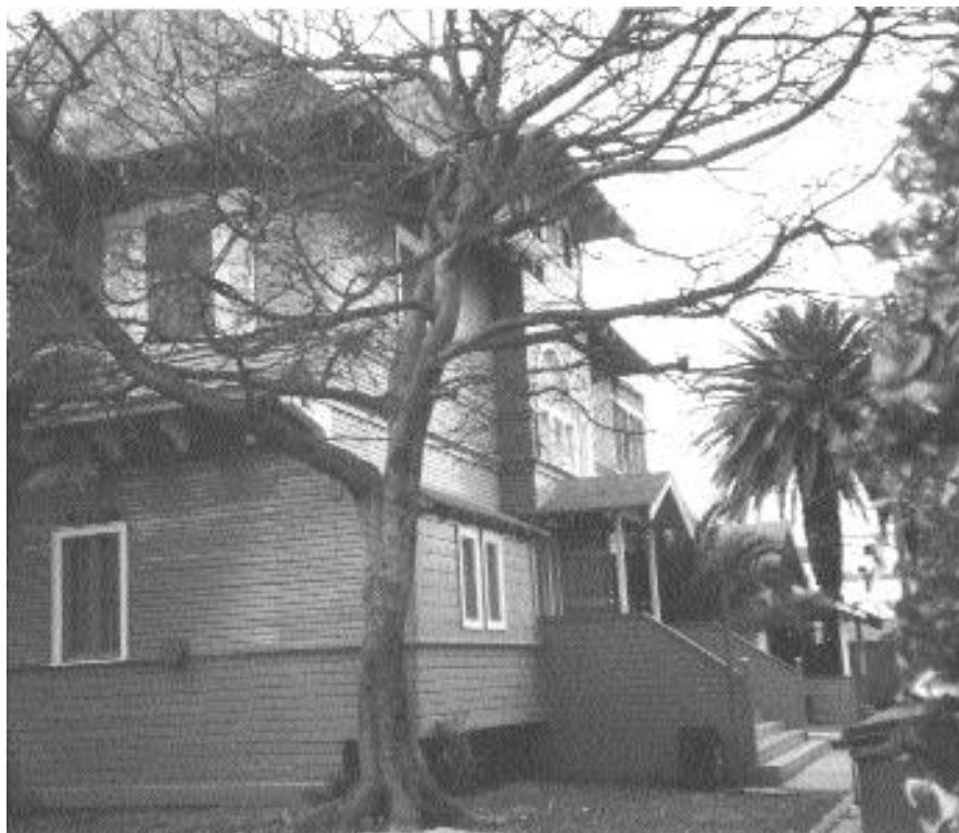
View of facade of 2701 Menlo Avenue
